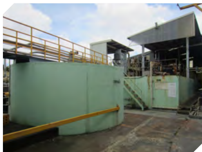
San Shing's pickling wastewater treatment plant
